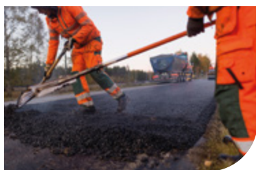
Construction materials and asphalt
